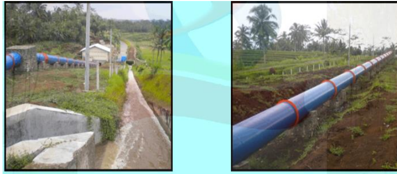
Gambar 2. 4 Pipa pesat (penstock)
