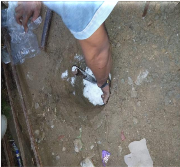
Gambar 16 (Menaburkan Garam NaCL 1 Kg)
