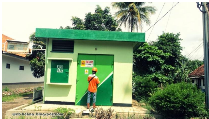
Gambar 2.5 Gardu Beton
