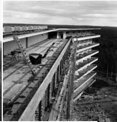
Gambar 3.8, Struktur Kantilever Sumber : kvadratinterwoven.com/paimio-sanatorium
