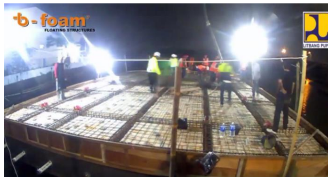
Gambar 2.5 Pengacoran lantai Sumber : https://www.youtube.com/watch?v=K9JcB7ybsIc
